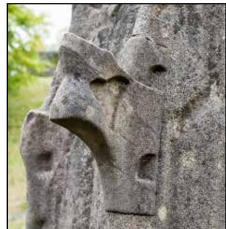
Differential weathering between the pinnacle and an earlier repair using an unknown stone.
